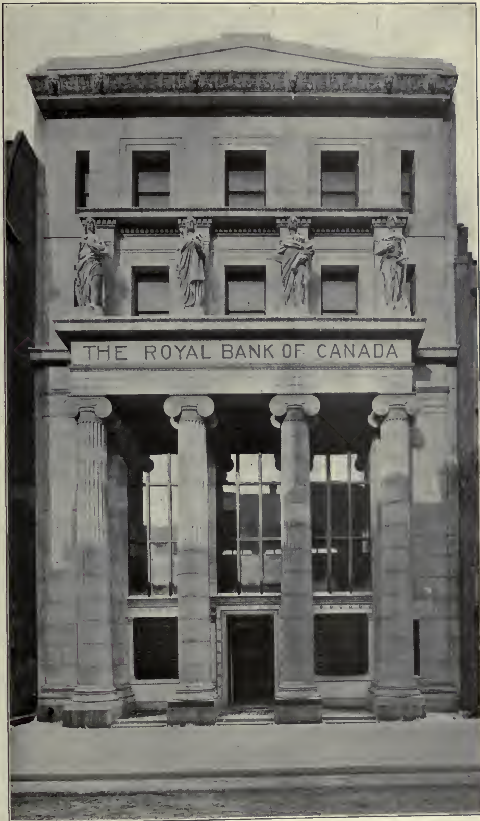
The Royal Bank of Canada, Head Office, St. James Street. Established 1869. The third largest bank in Canada. Capital Paid Up, $11,560,000; Reserve, $13,000,000, and Assets $175,000,000. This building in process of enlargement.
